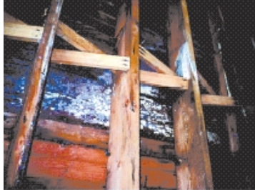
Heavy mold growth on underside of spruce floorboards.
