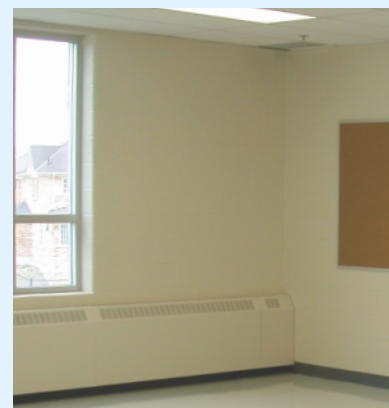
Masonry wall construction in public buildings reduces the likelihood of mold growth.
